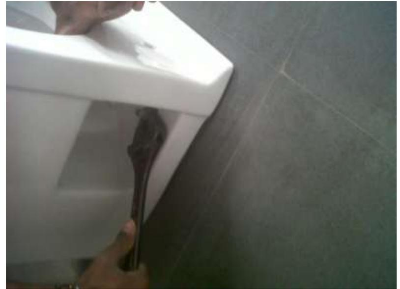
**Screw in washers and nuts into the rag-bolts. Tighten with spanner.**
