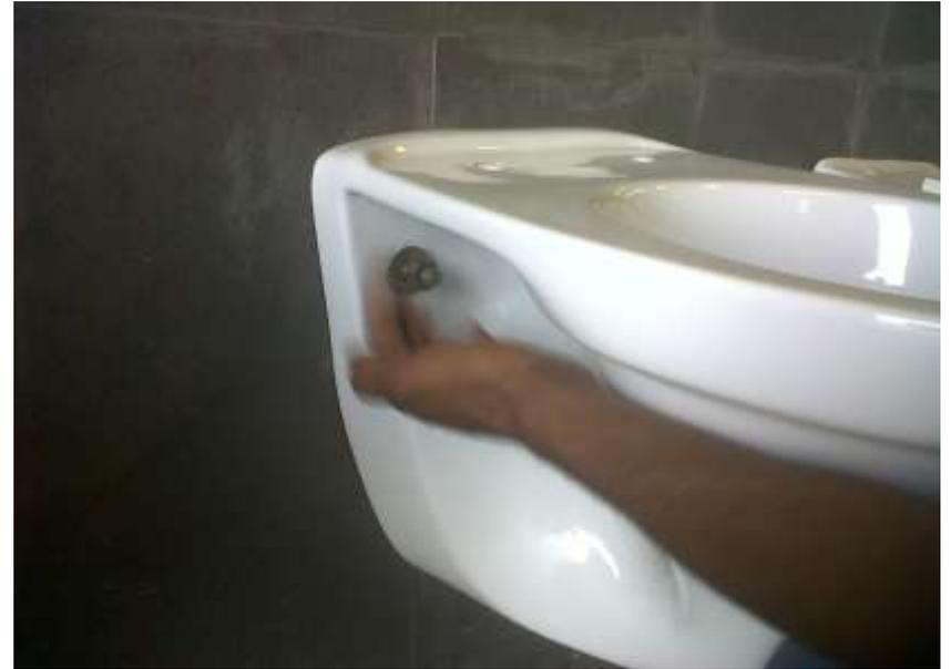
**Insert the washers and nuts into the rag-bolts as illustrated.**
